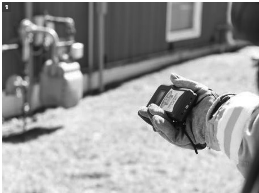
(1) A firefighter points the handheld laser gas detector at a commercial meter to determine if gas is leaking. (Photos by author unless otherwise noted.)
