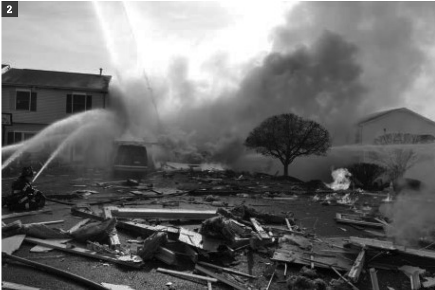
(2) In 2012, an underground gas leak migrated into a nearby home and subsequently exploded, nearly killing the author and another West Haverstraw (NY) firefighter. (Photo by Dom D'Alisera.)
